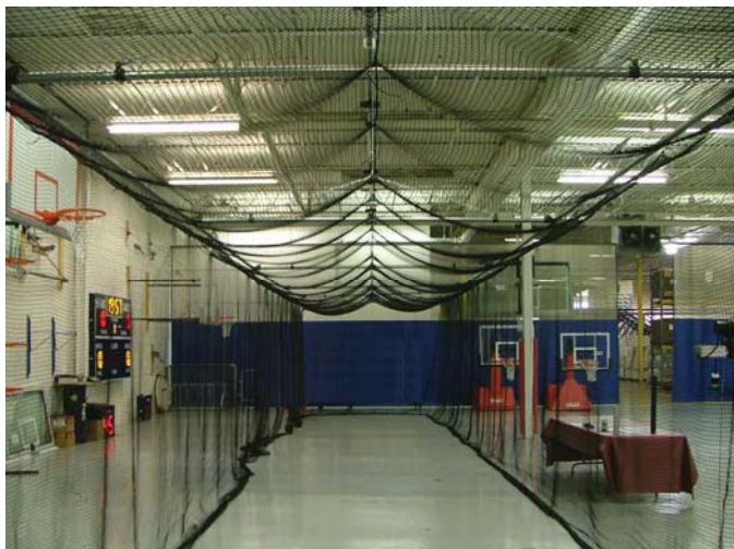
Interior view of cage with netting being picked up at both ends of frame and at the center cage tension cable.
