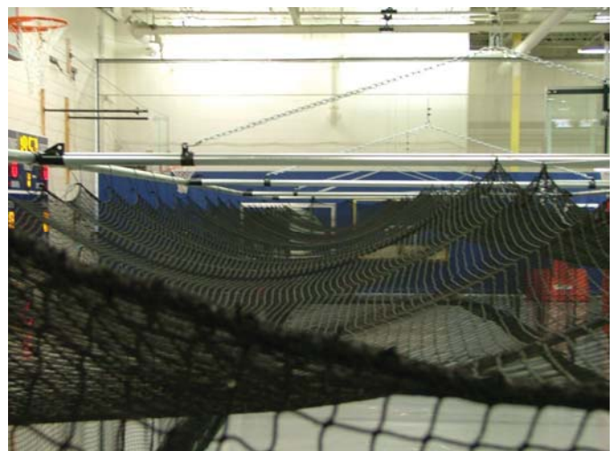
Top netting attachment detail showing 6" nylon tie drop at side frame and center cage tension cable.
