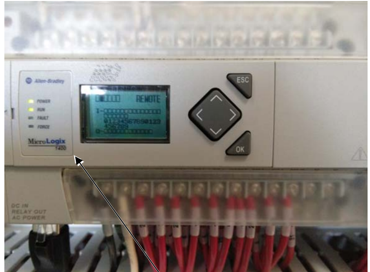
MicroLogix 1400 PLC in Powr-Touch 5.0 panel
