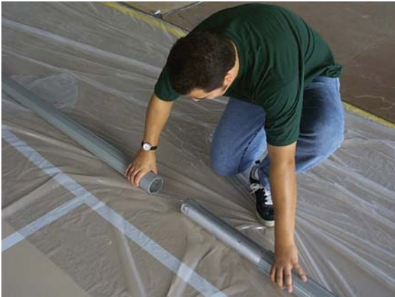
Connecting Batten Tubes at Splice Location
