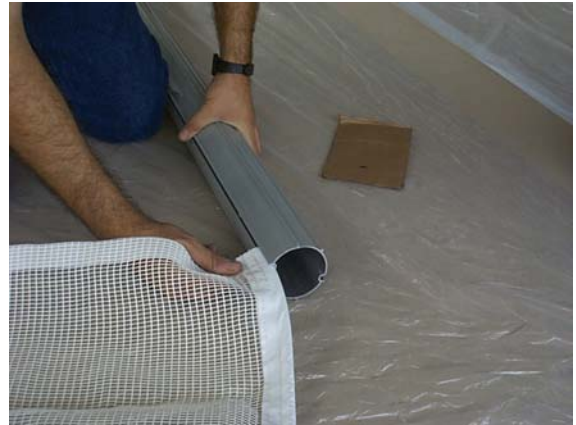
Sliding Fabric Panel into Batten Tube Cable Slot
