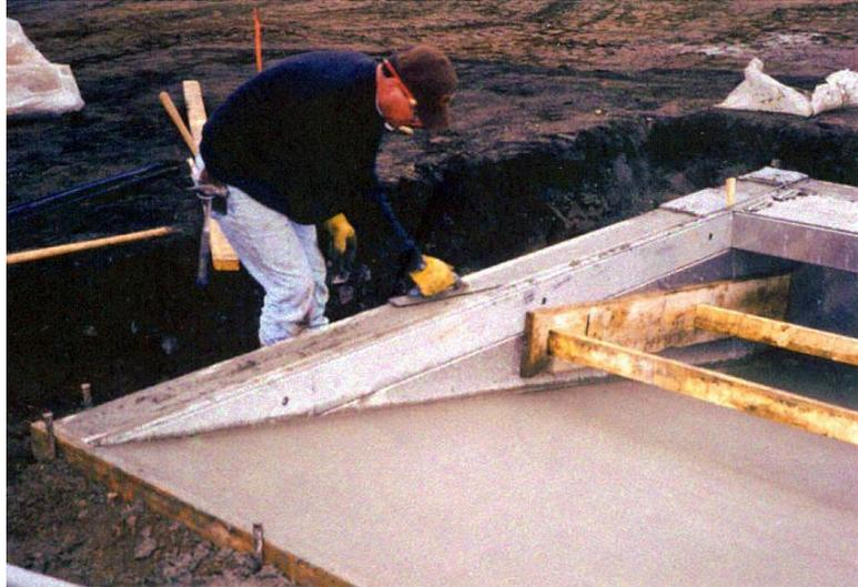
Pour concrete into form and level off. Use ledges on the side walls and front wall to level off the floor.
